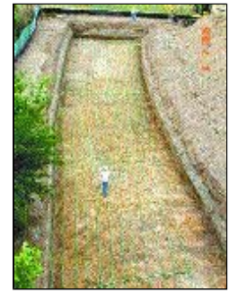
Installing looped piping.
