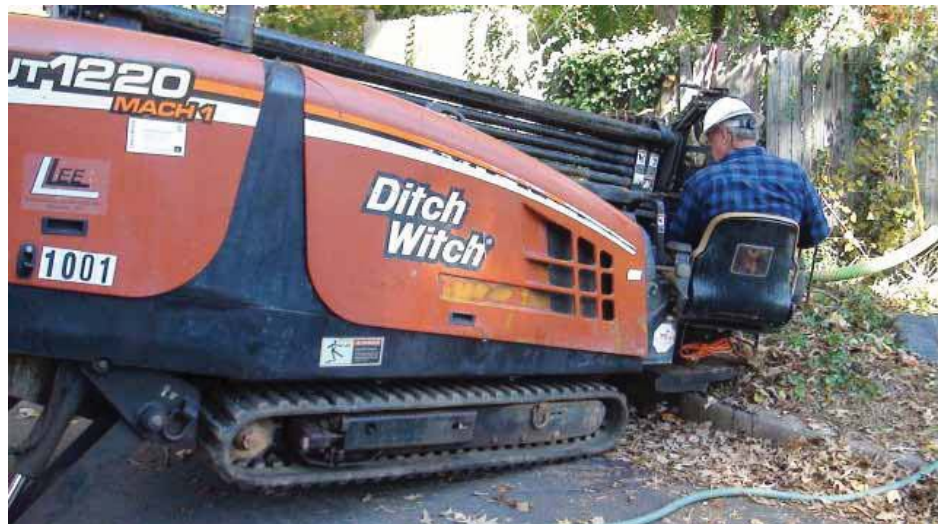
Lee Electric on the job.
